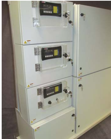
Custom designed modular cryo storage: Control/power and high stage compression module.
